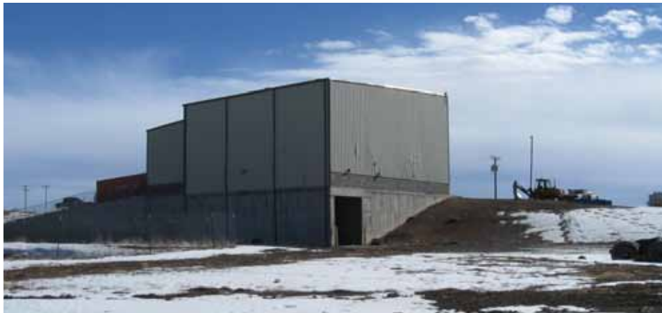
Exhibit VII-2 Solid Waste Facility
